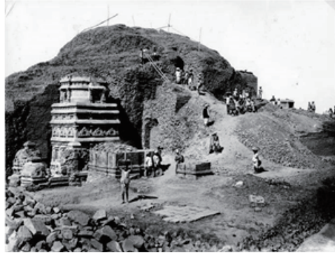
Photograph of excavations in progress at Nalanda, Marshall Collection (DUROM.1957.1.3365)
